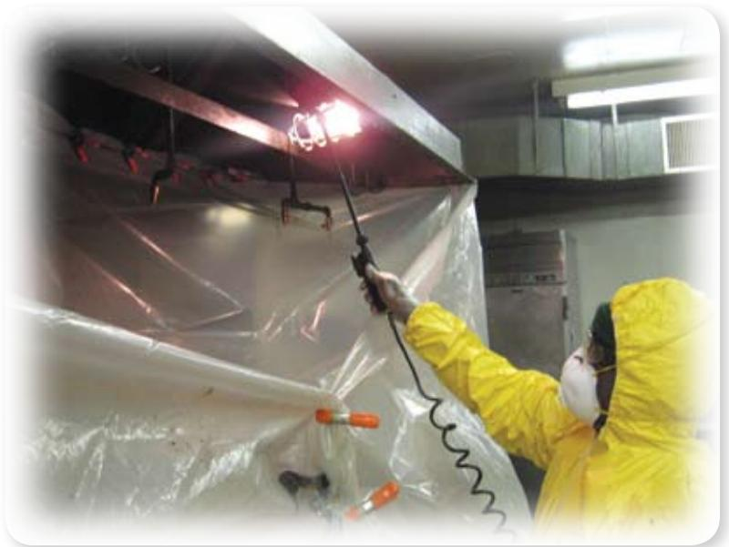
Fiberglass extension ladders for access to the roof and fiberglass A-frame ladders for the interior work are necessary. Fiberglass extension poles with magnetic scrapers will be required in order to properly remove grease and particulate build-up from the exhaust shafts and ductwork.
